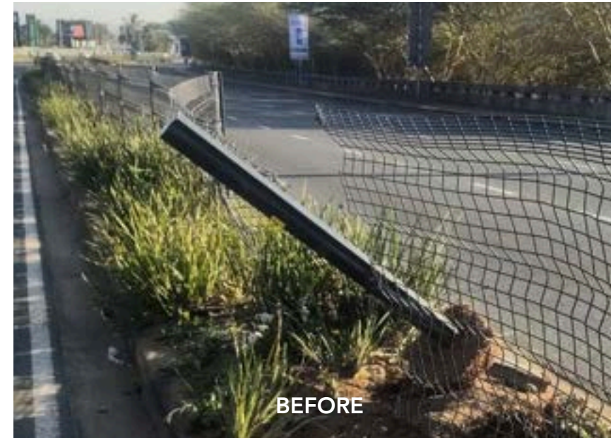
P445 Fence Repairs
