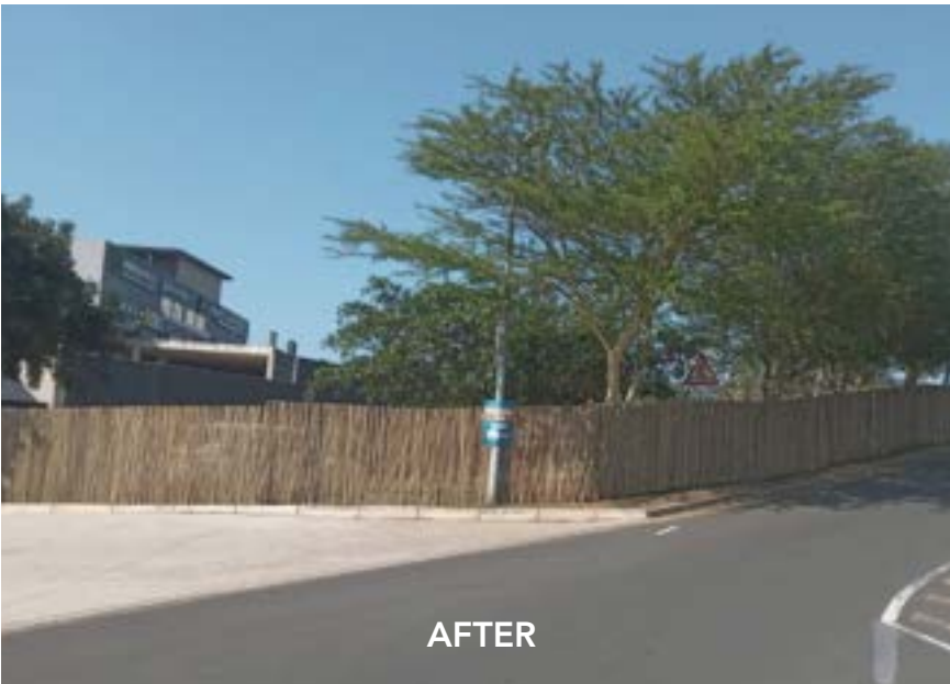
New Uber Parking Fence Installation
