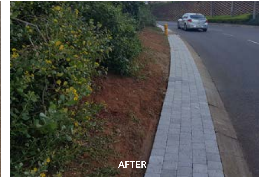
Douglas Crowe Pedestrian Paving Installation
