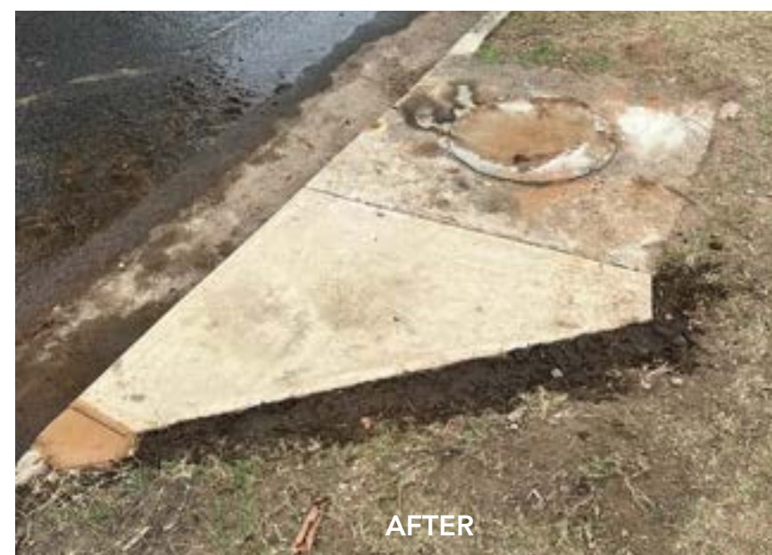
Stormwater Drain Repair
