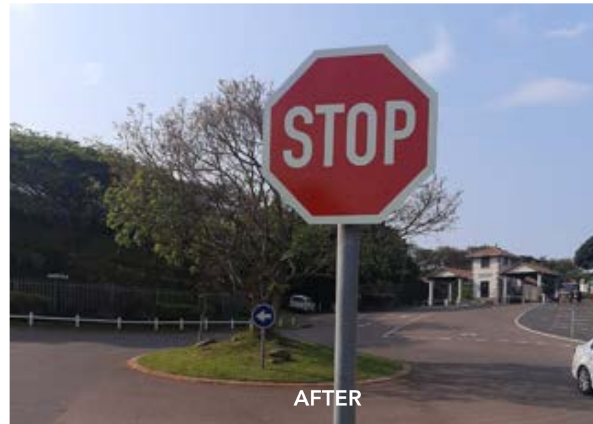
Traffic Sign Replacement
