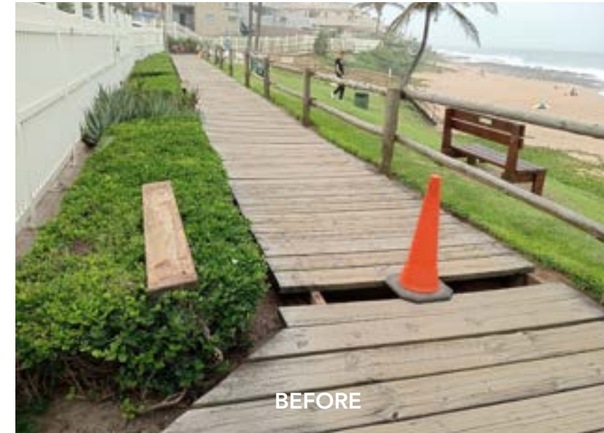
Promenade Plank Repairs
