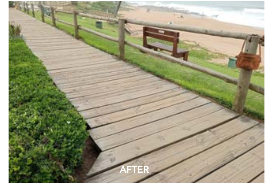
Promenade Plank Repairs
