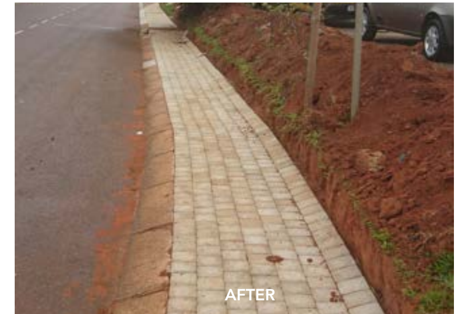
Business Park Pedestrian Walk Paving Installation
