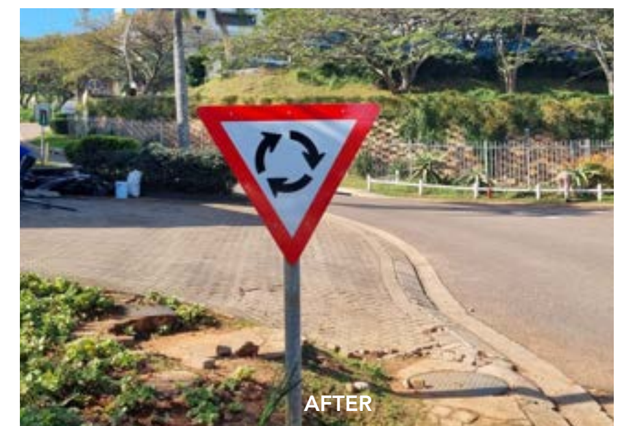
Traffic Sign Replacement
