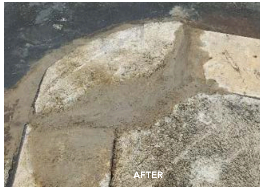
Leonora Drive Paving Repairs
