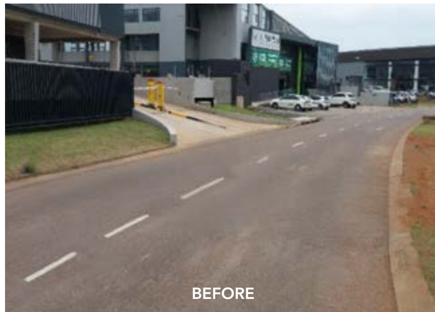
Business Park Speed Hump Installation
