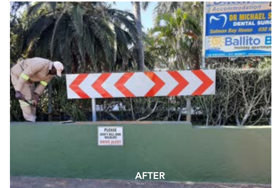
Chevron Board Replaced
