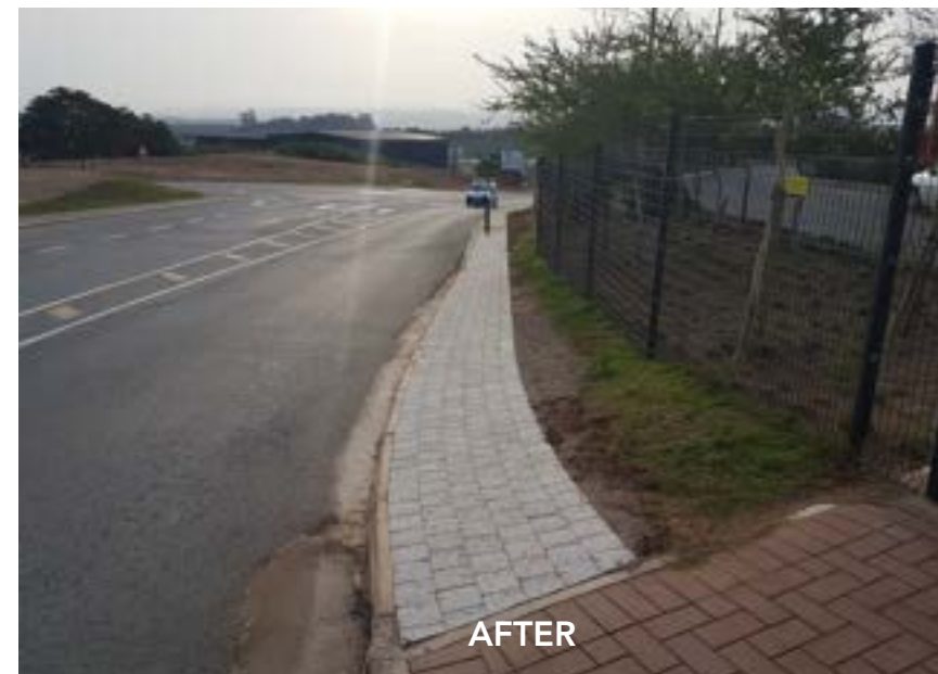
McDonalds Verge Paving Installed
