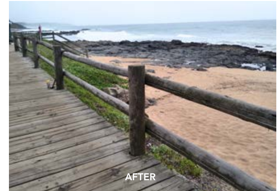
Post & Rail Repair
