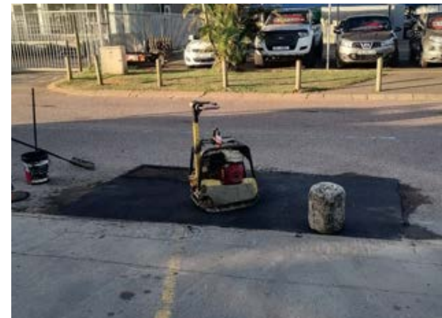
Ongoing Pothole Repairs
