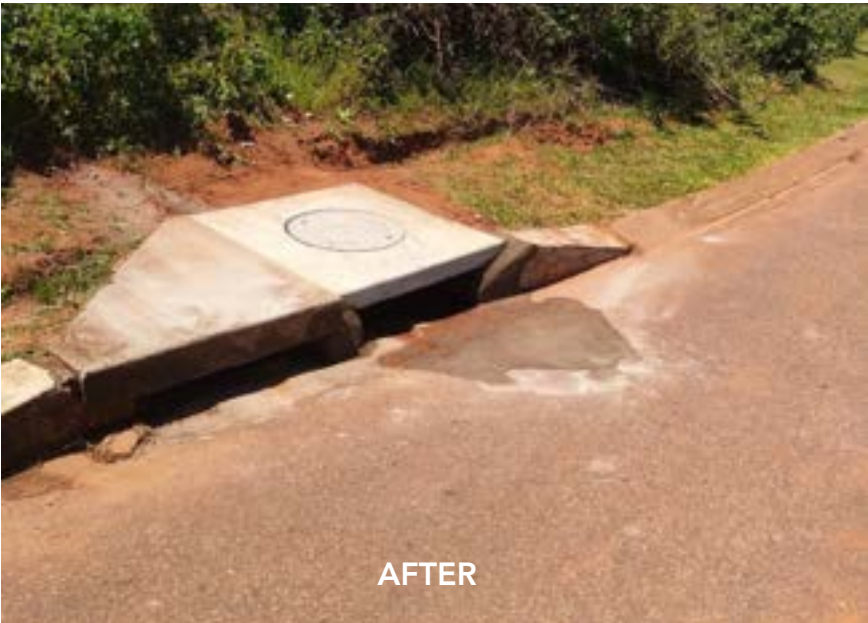
Catchment Cover Replaced
