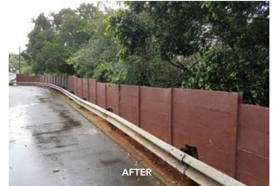
Ballito Drive Wall Revamp
