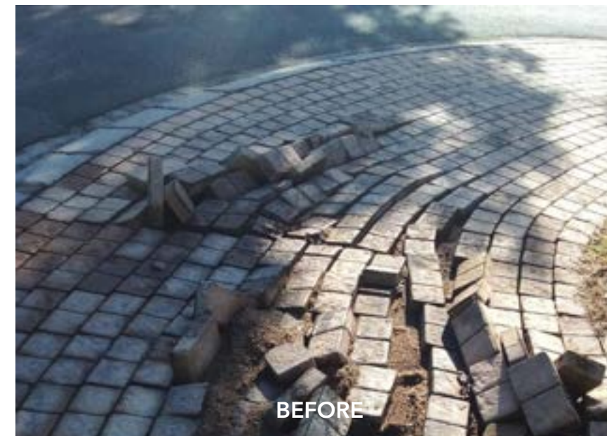
Traffic Circle Paving Repairs
