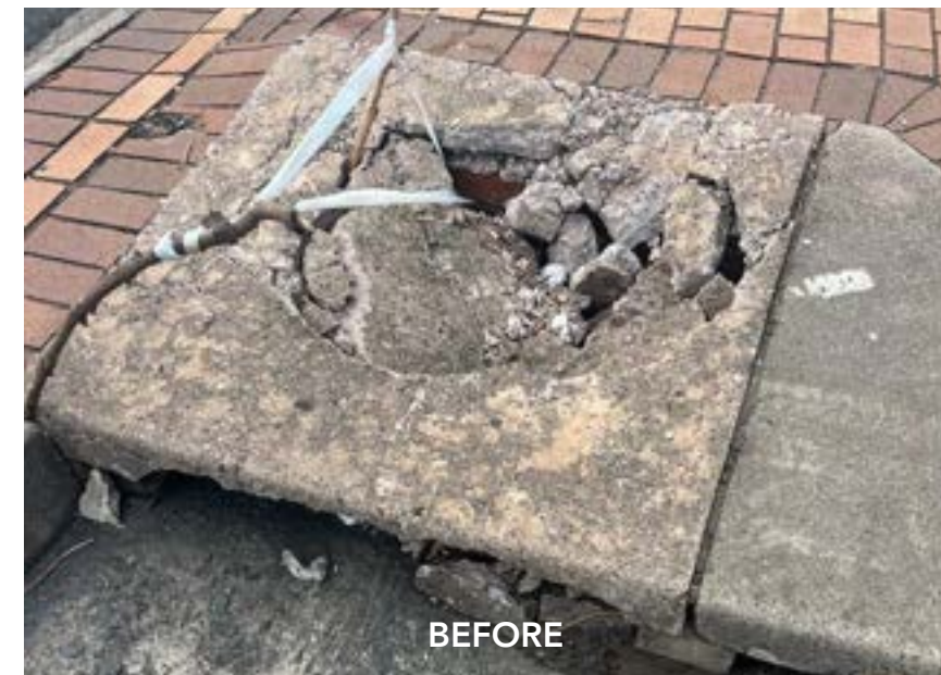
Storm Water Drain Repairs
