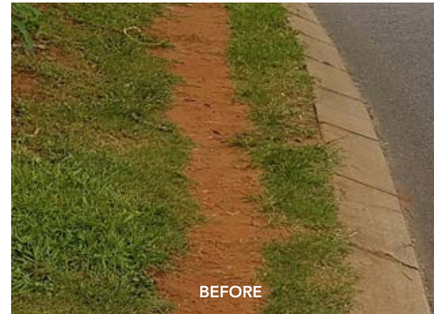
Douglas Crowe Pedestrian Paving Installation
