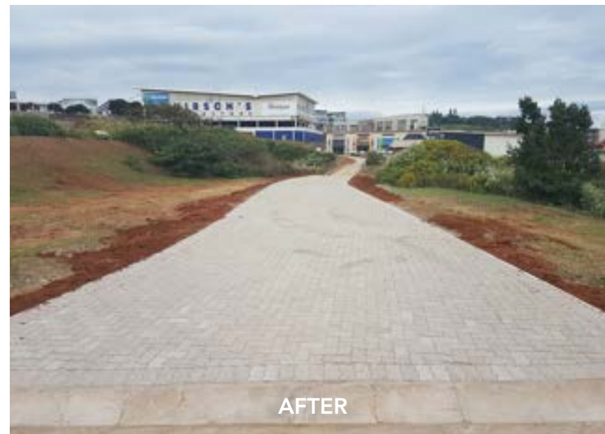
Agricultural Bridge Paving
