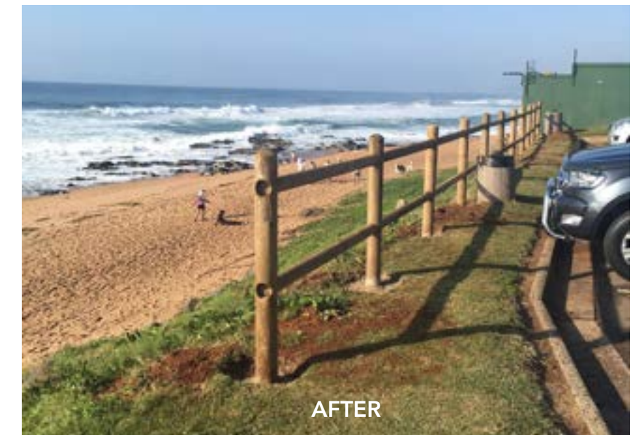
Foch Le Roux Fence Installation
