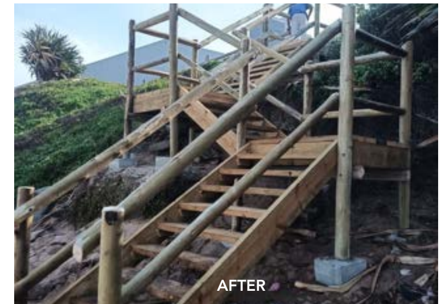
Promenade Staircase Replacement
