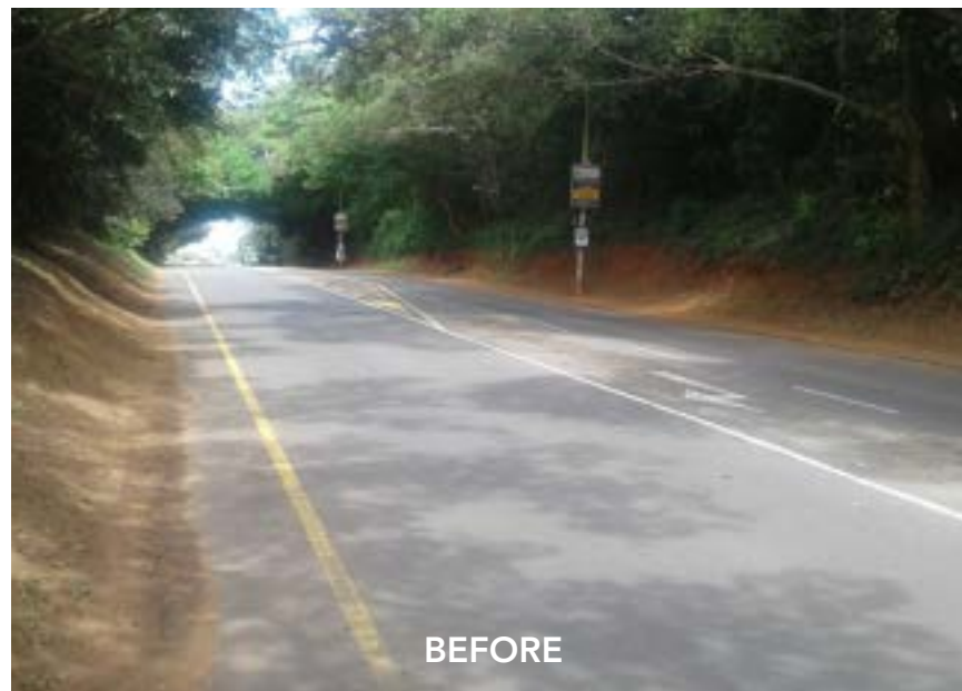
Ballito Drive Dianella Installation
