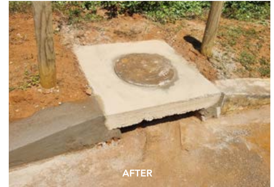
Stormwater Drain Repair
