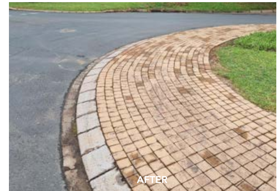
Traffic Circle Paving Repairs
