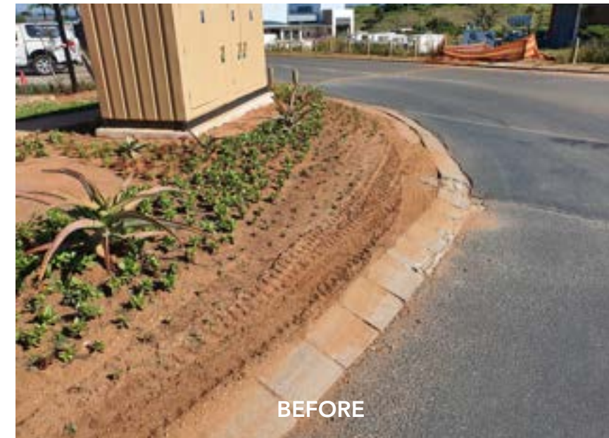
Moffatt Road Corner Repairs
