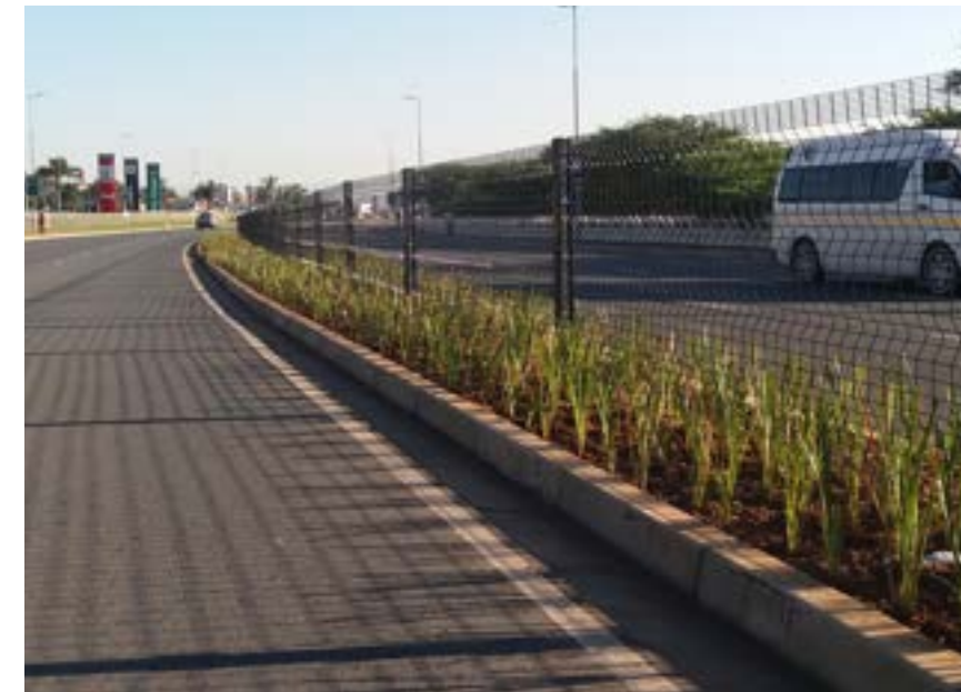
P445 Fence Installation
