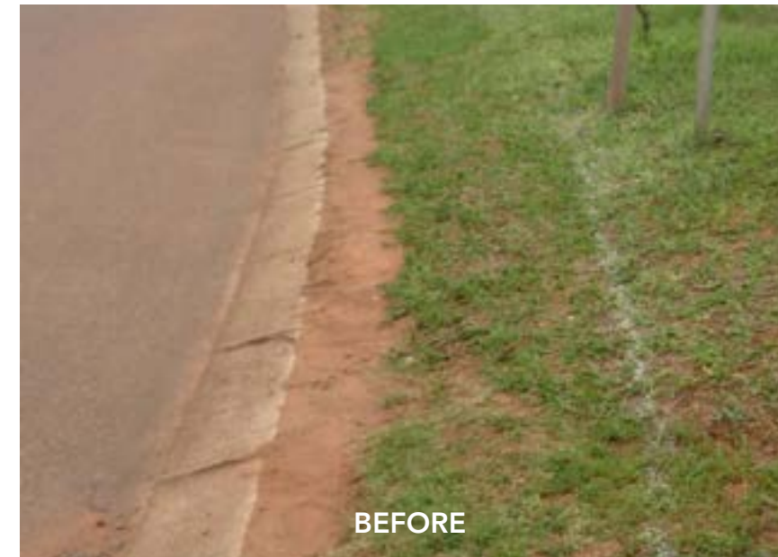
Business Park Pedestrian Walk Paving Installation
