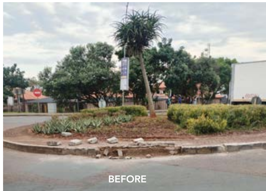
Traffic Circle Upgrade
