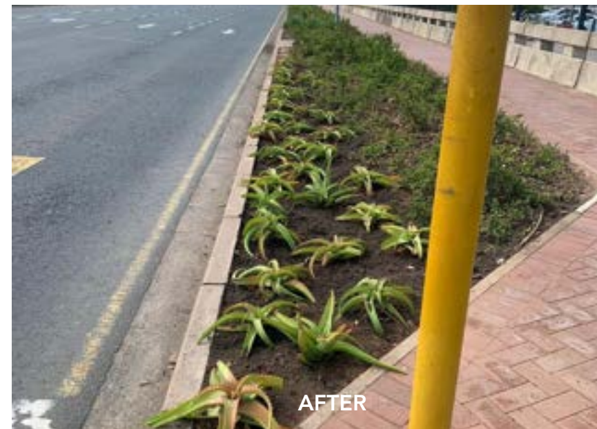
P445 Landscaping Upgrades
