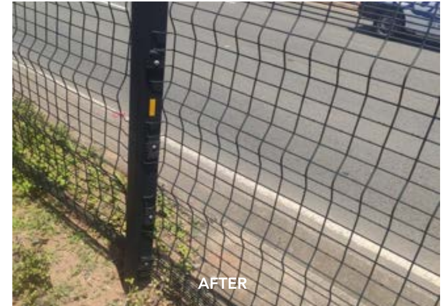
P445 Fence Repairs
