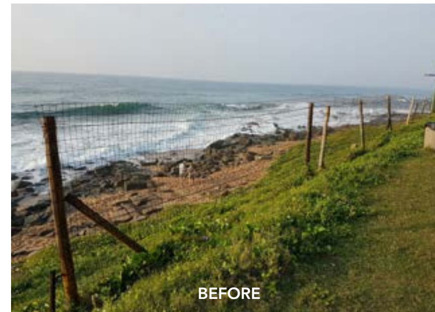
Foch Le Roux Fence Installation
