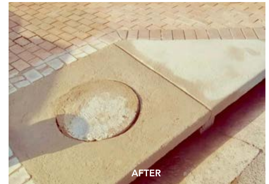
Storm Water Drains Repairs
