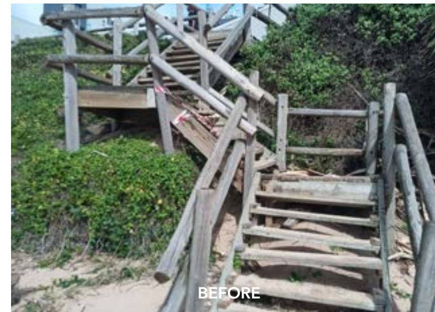
Promenade Staircase Replacement
