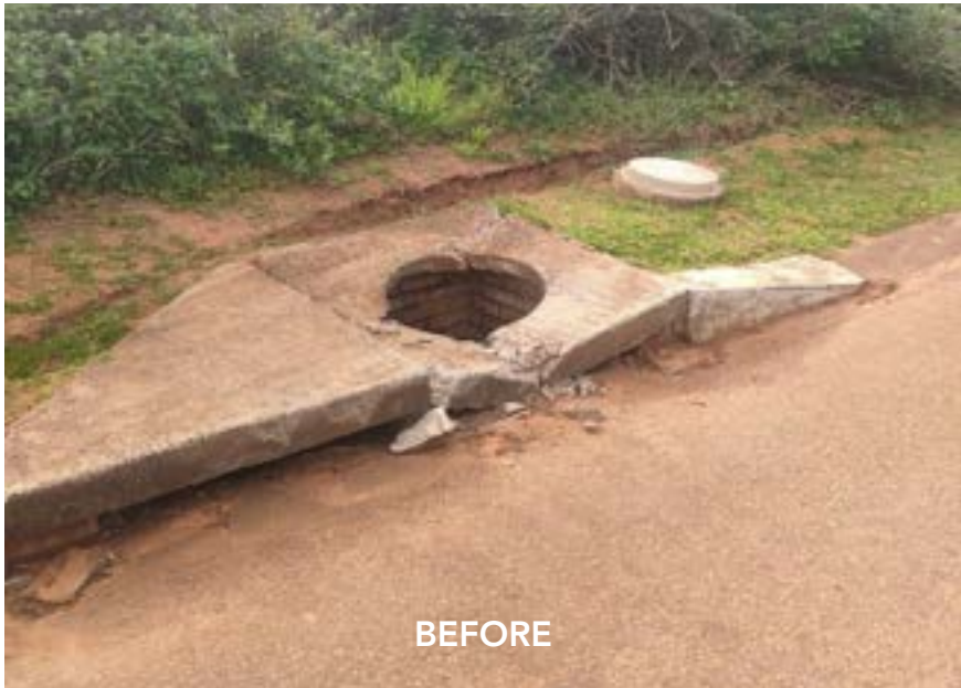
Catchment Cover Replaced
