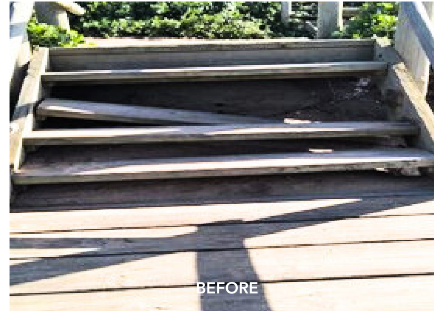
Promenade Stair Repairs
