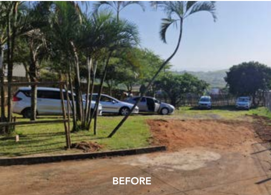
New Uber Parking Fence Installation
