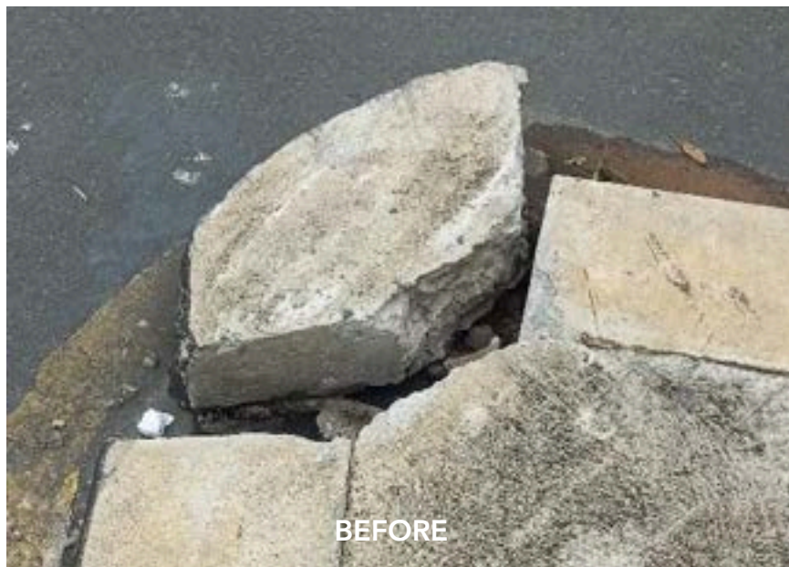
Leonora Drive Paving Repairs
