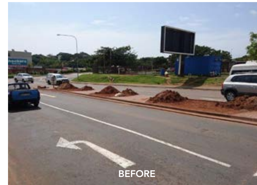
Centre Median Paving Removal
