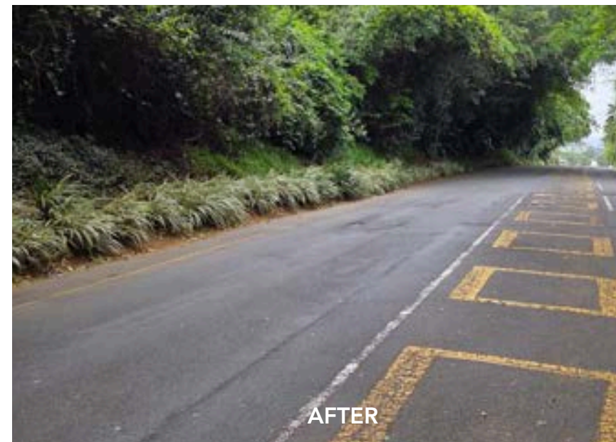
Ballito Drive Dianella Installation
