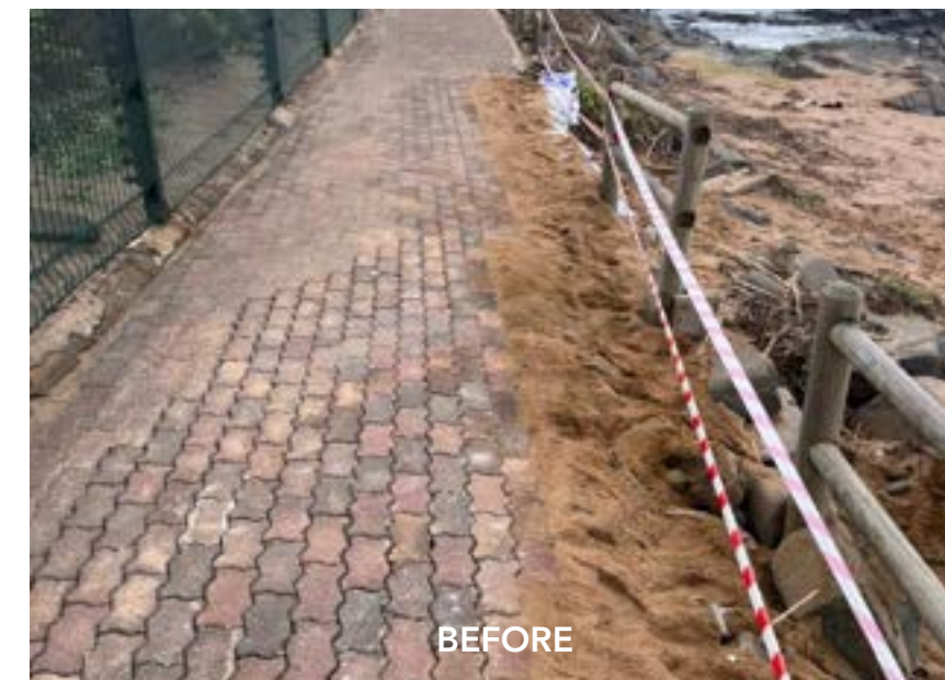
Promenade Post Storm Repairs
