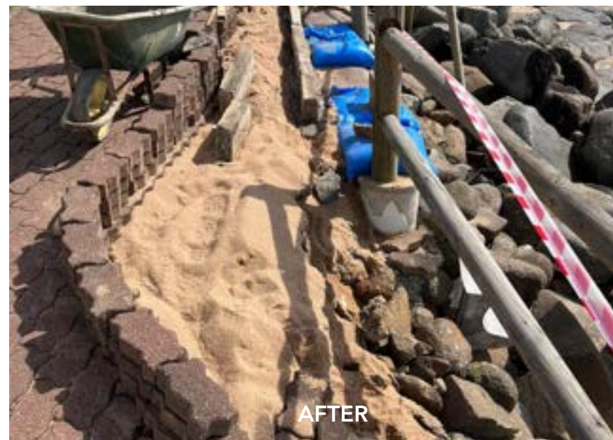
Promenade Post Storm Repairs
