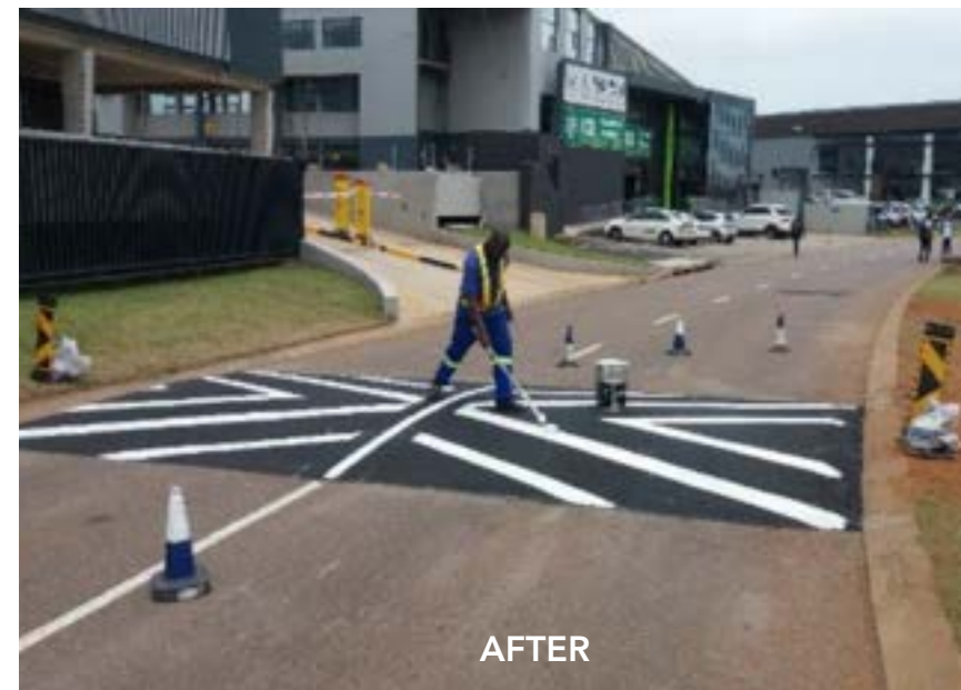
Business Park Speed Hump Installation
