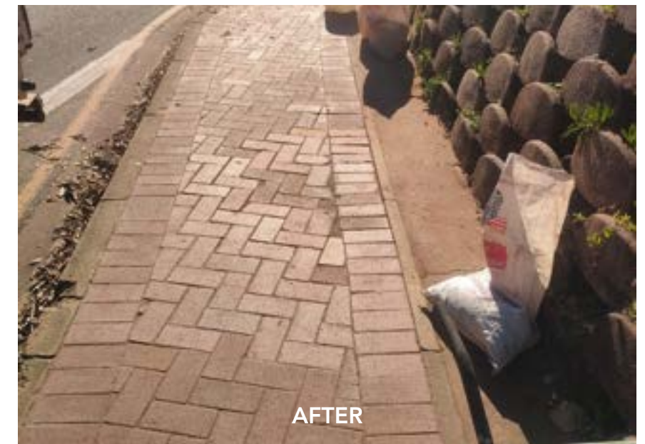
M4 Paving Repairs
