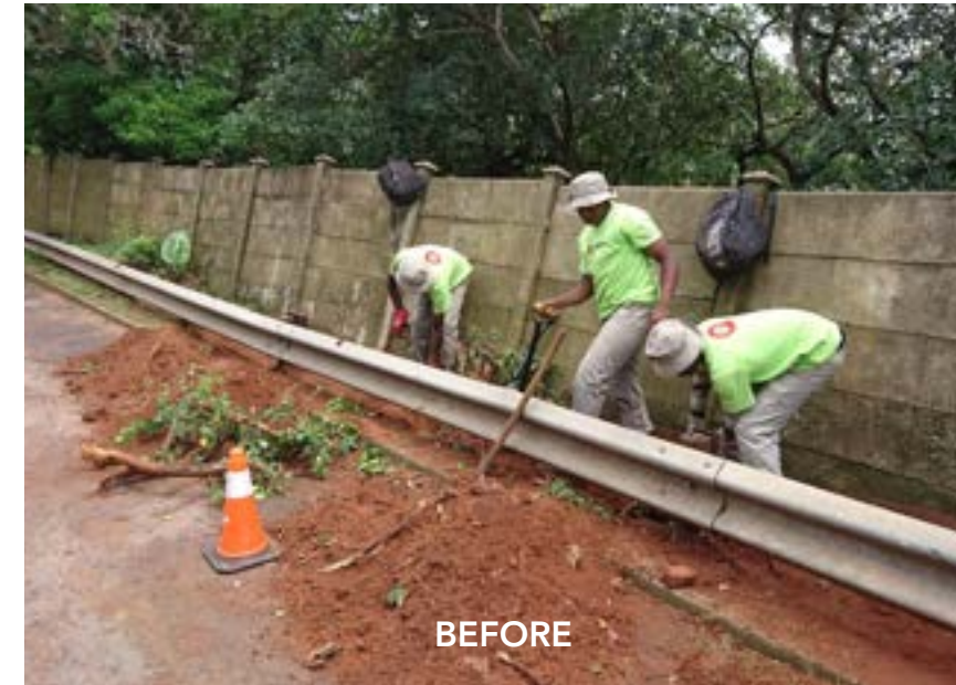
Ballito Drive Wall Revamp
