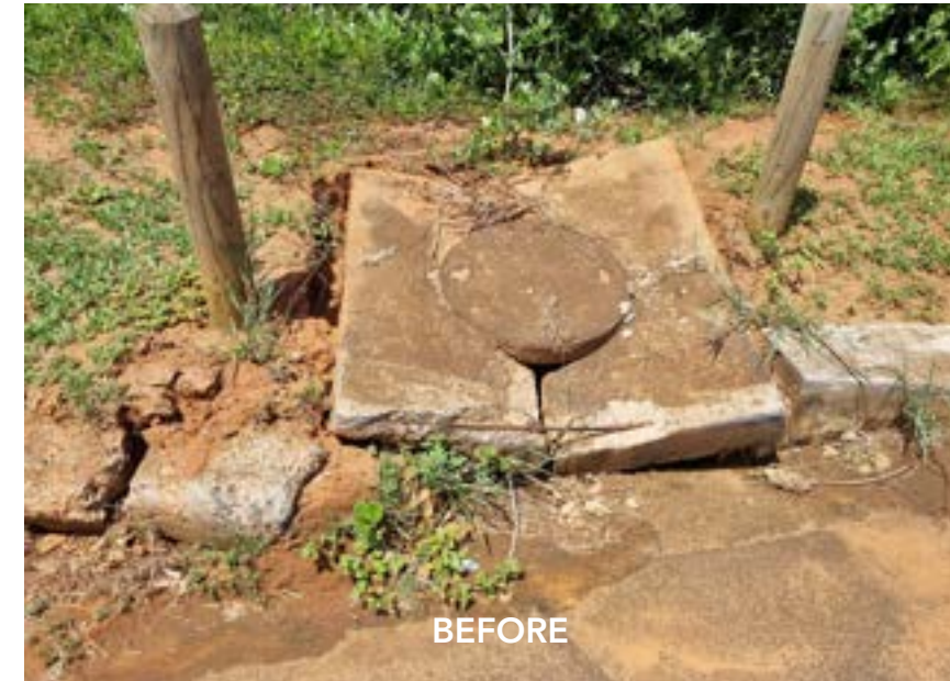
Stormwater Drain Repair
