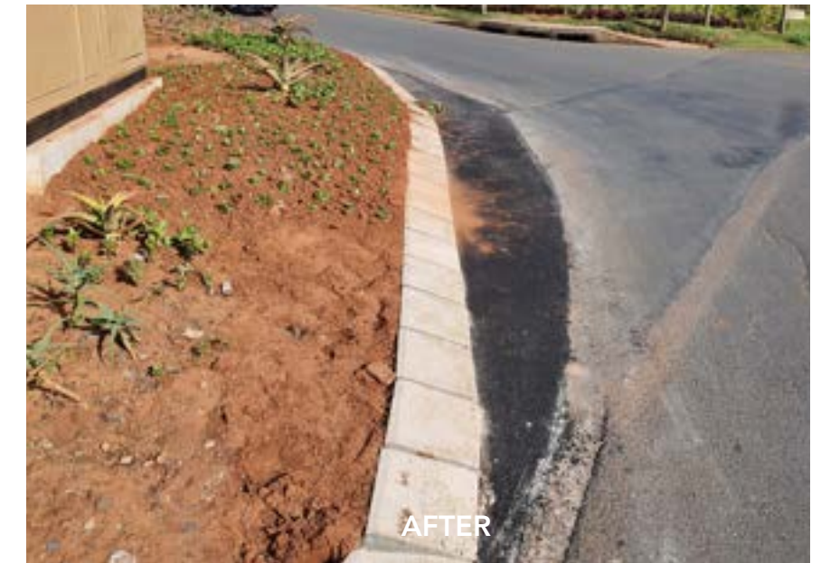
Moffatt Road Corner Repairs
