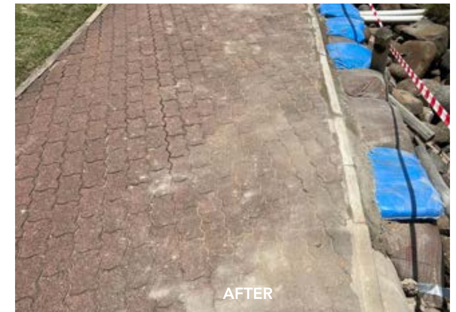
Promenade Post Storm Repairs
