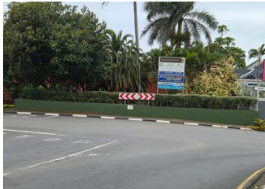
Ballito Drive Wall Revamp
