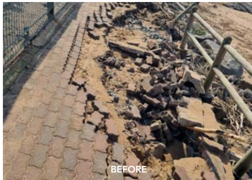
Promenade Post Storm Repairs
