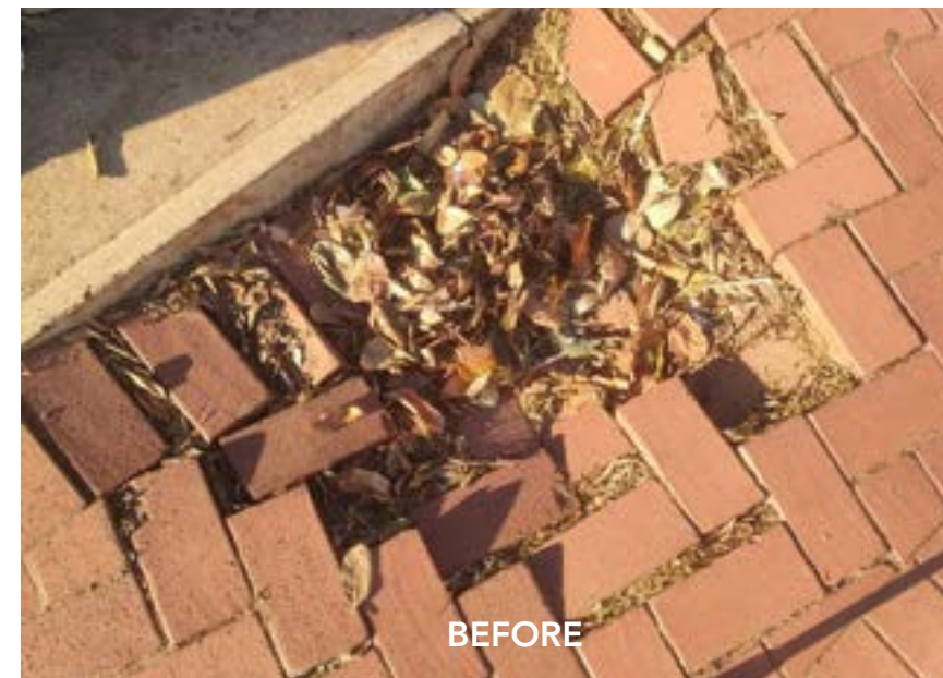
M4 Paving Repairs
