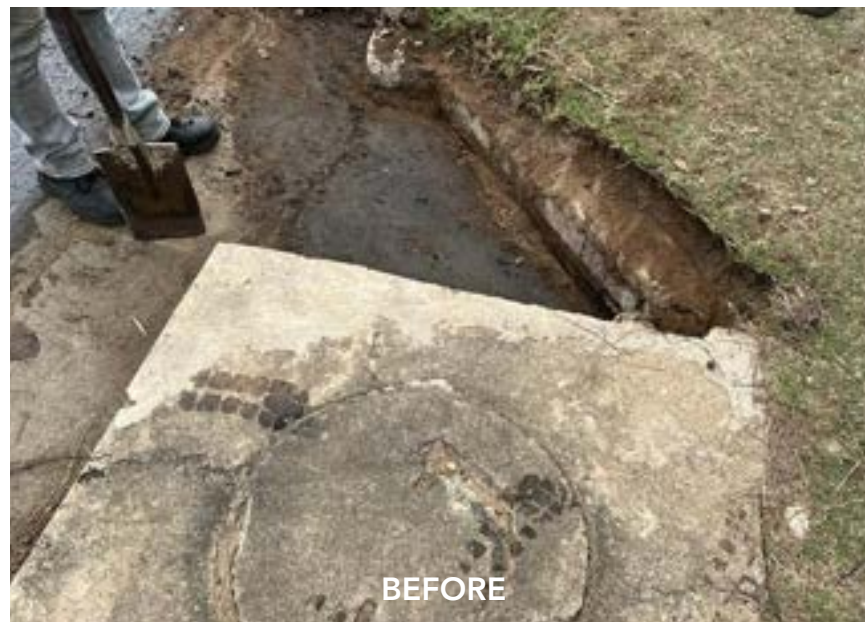
Stormwater Drain Repair
