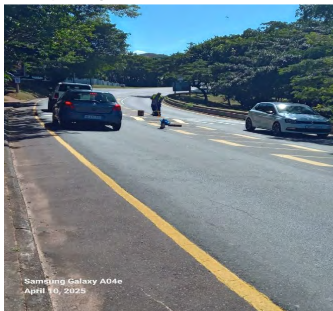
KDM painting traffic lines in the Business Park
